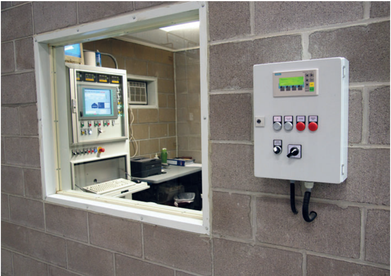
Fig. 5: The ACT SmartTouch control is a PC-based PCS Control System situated in an unattended control room. The PCS control produces precision concrete for high output quality SCC concrete. A simple remote call station is mounted by the mixer platform and is the only interface the crane operator needs to call a batch of concrete. The user-friendly PCS control records every batch for quality assurance and easier inventory accounting. Hydromat mixer-mounted microwave moisture probe and Hydrotester aggregate bin moisture sensors provide real-time water/cement ratio adjustment for SCC accuracy.
